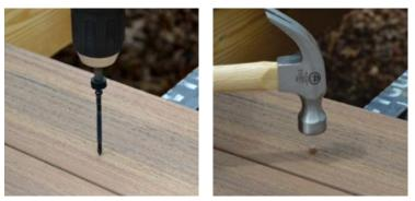
A special driving tip automatically puts the Cortex® screw at a precise depth. Then, the color-matched plug is tapped in with a hammer.
